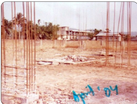
Completion of Pilings in April, 2004
