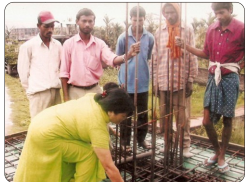
(Lt.) Pi. Ngailhing Haokip taking part in slab casting
